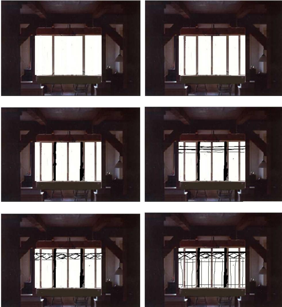
*Sequence Of Surveyor's tape mockups Generating The Form Of The Window By Morphogenesis*
