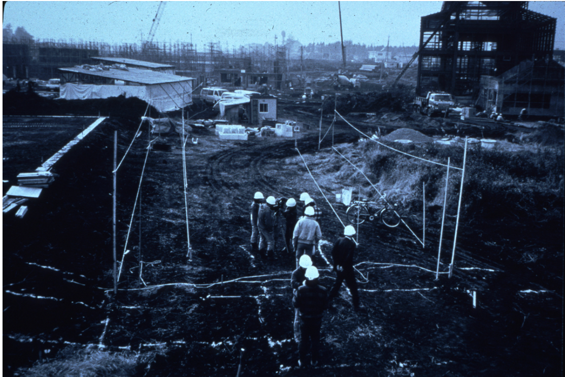
Modifying stakes to mark the entrance street, once the volume of the great hall was in place, and allowed us to make more accurate judgments about the angles and positions of the street and its edges.
