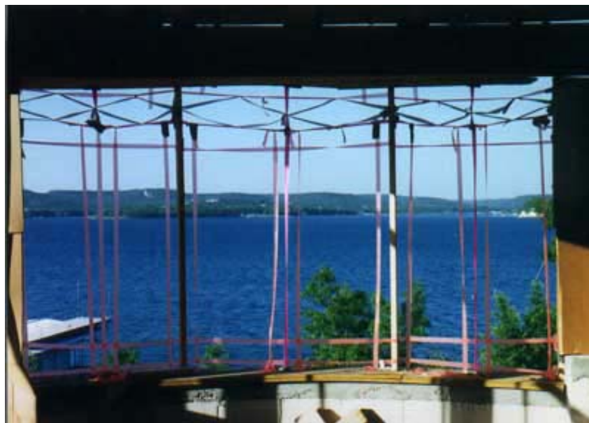
Final surveyor's tape mockup for the window in the Gioja house
