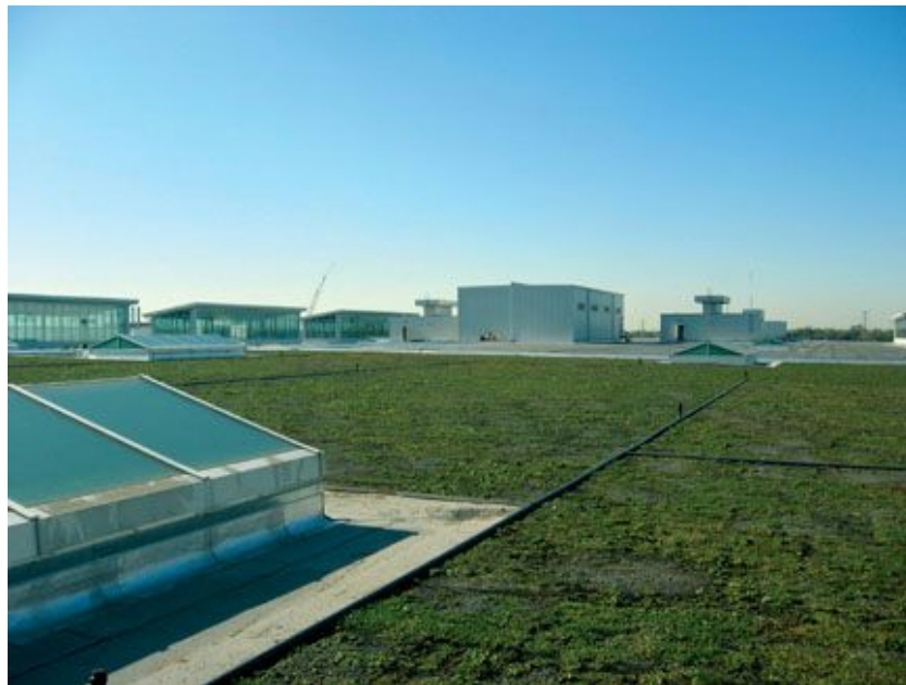
Grass on the rooftop of the Ford plant, William McDonough
