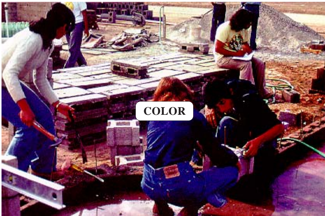
Our manufacture of special interlocking earth-cement blocks designed to be placed in a way that allows unfolding to proceed smoothly and without backtracking.
