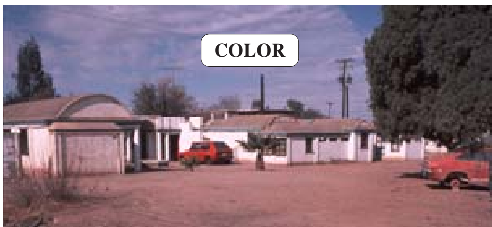
A part of the community of houses built using this technique of unfolding. Without introducing any additional construction cost, each house turns out unique and different according to its situation.
