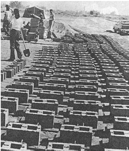
Foundation blocks after molding curing in our yard.
