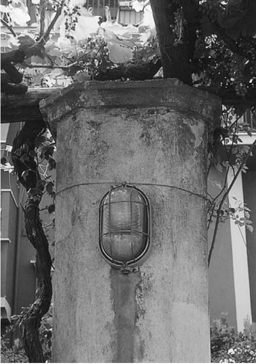
Light placed to help the top of the column
