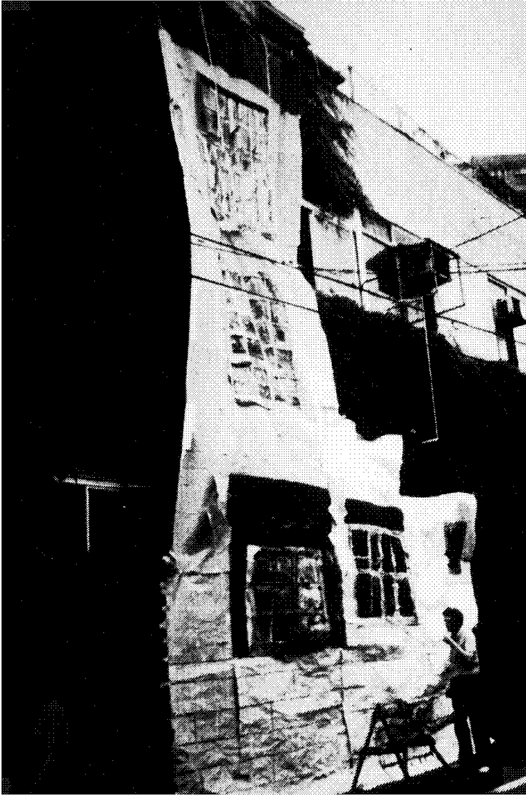
Emoto building, Tokyo. The picture shows Hajo Neis making a fullsize mockup in painted paper on the building that existed previously on the site, to study the effect of the elevation design and materials on the street, so that we could make sure that the street was helped by the building
